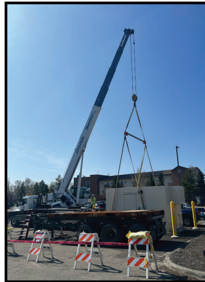
JBER Back-up Generator Installation
