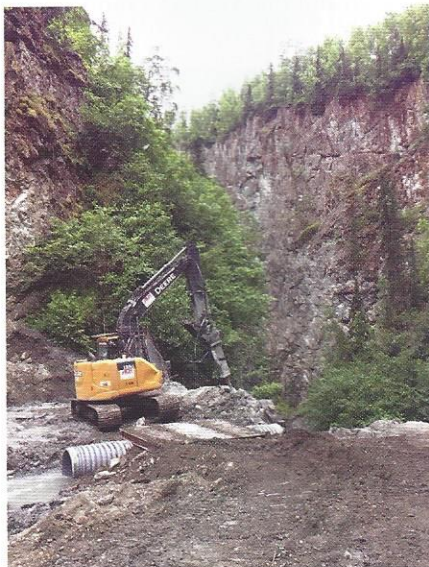
Hydraulic hammering of the concrete to demolish the dam.
