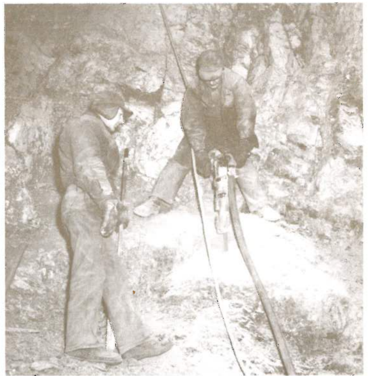
Drilling holes for blasting charges in tunnel
