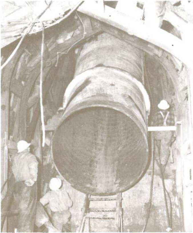
Installing penstock pipe, 1954
