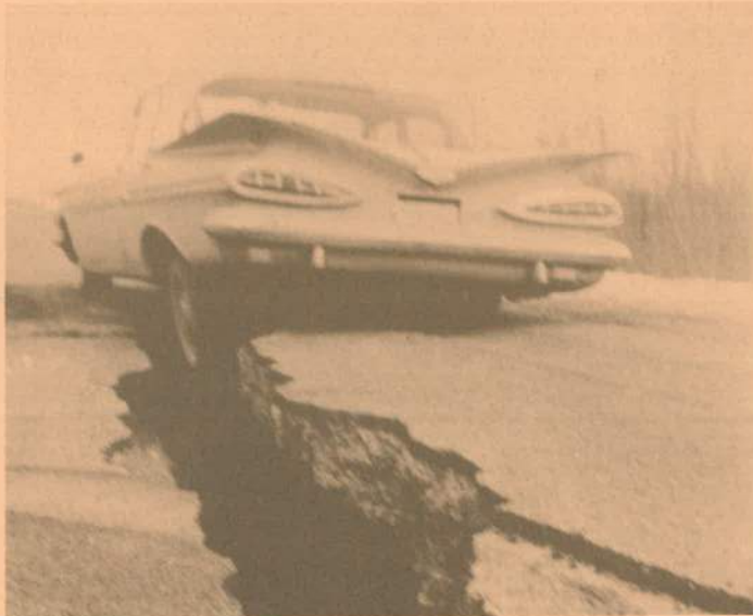
Earthquake damage to highway near powerplant
