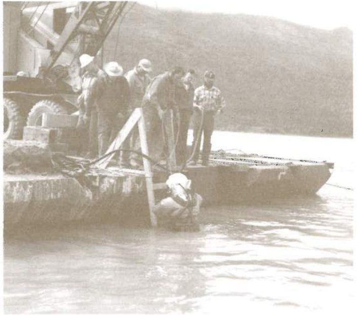
Diver working during excavation for intake structure on Eklutna Lake bottom
