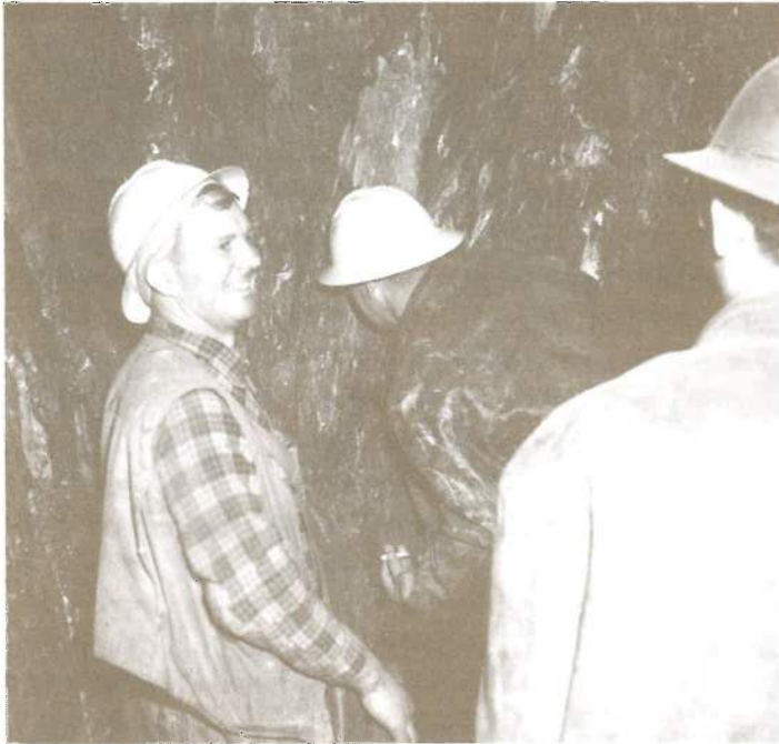
Engineer peering through hole between north and south tunnel headings, October 15, 1953
