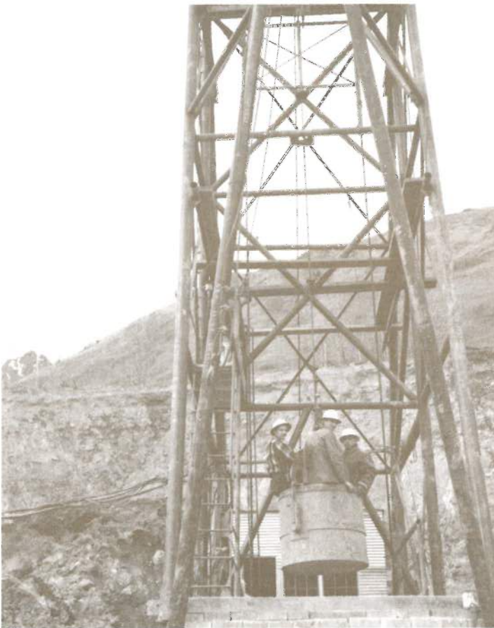
Workmen being lowered into tunnel gate shaft, June 1952
