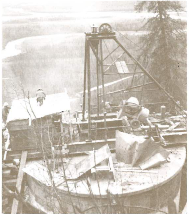
Winch headframe and workmen completing construction of surge tank, fall 1954
