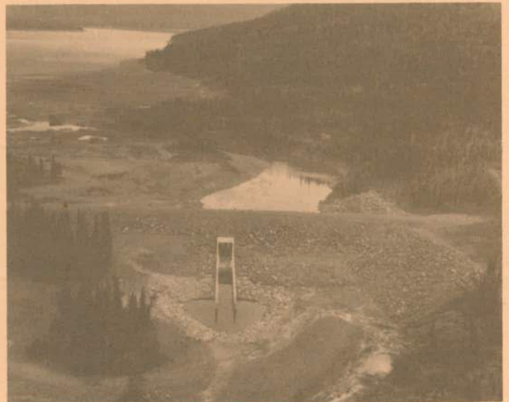
Eklutna dam, constructed 1965. Remains of old dam are above the new dam, at left edge of photo.
