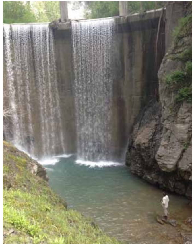
Lower Eklutna River Dam.
