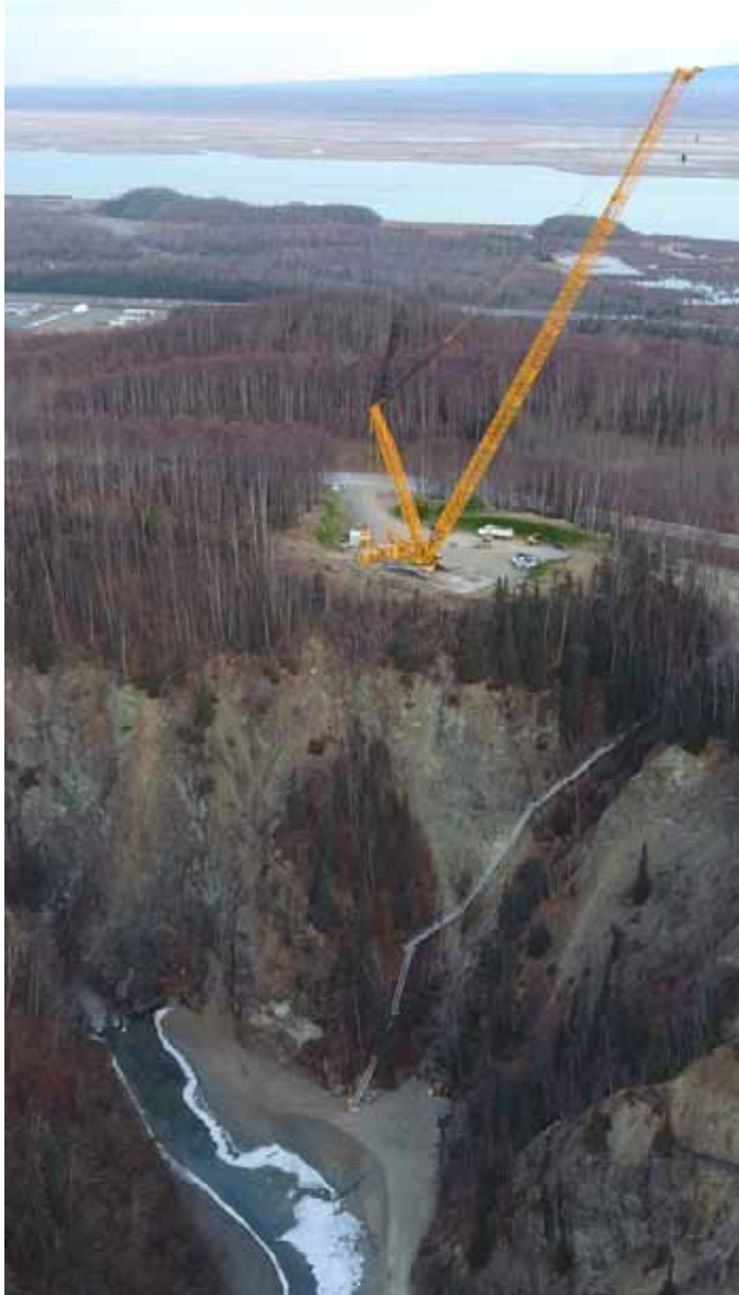
400-foot crane and staircase into Eklutna canyon; native village of Eklutna in background.
