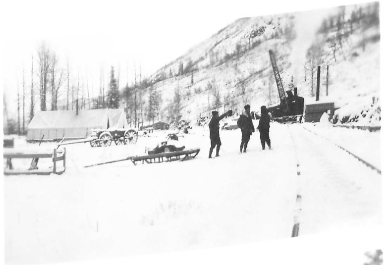
Figure 7 Power house site. Construction camp in foreground. Nov. 20, 1928
