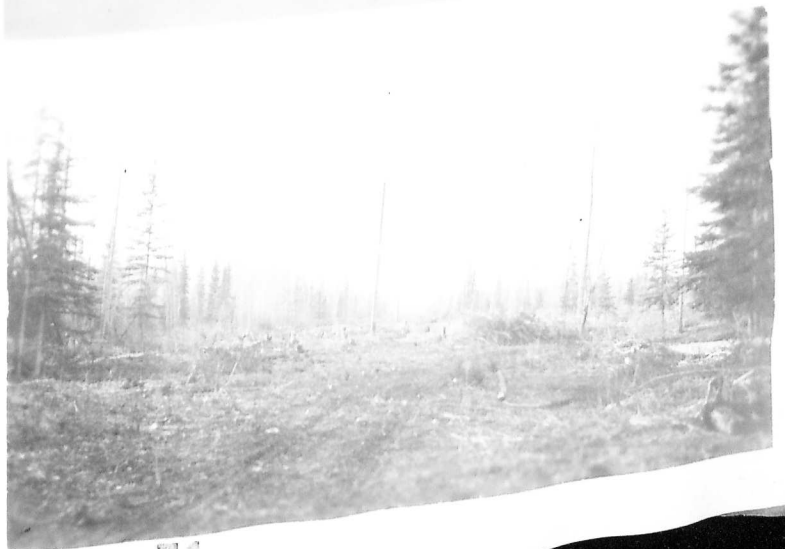
Figure 8 Anchorage transmission line under construc- tion. Oct. 30, 1928
